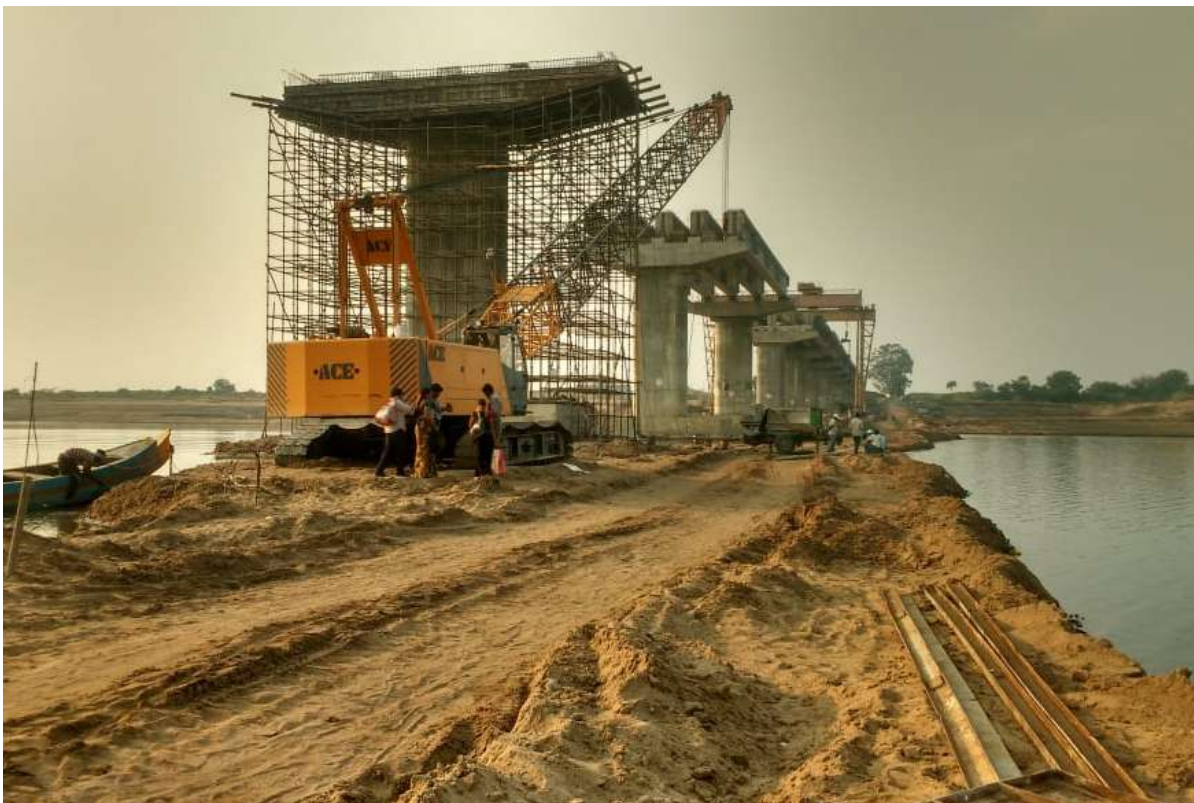
PSC GIRDER LAUNCHUNG AT PRANHITA SITE
