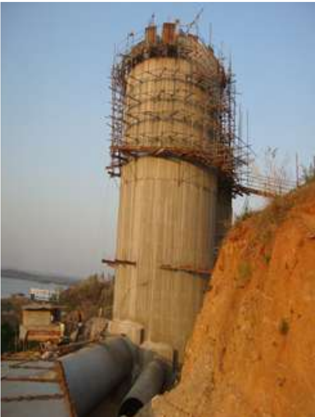
BREAK PRESSURE TANK (BPT) AND THRUST BLOCK
