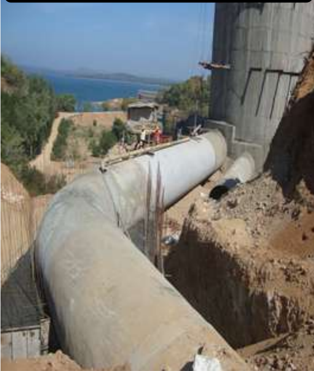
Thrust Block Construction executed under Supervision of Er. Anup Sangode
